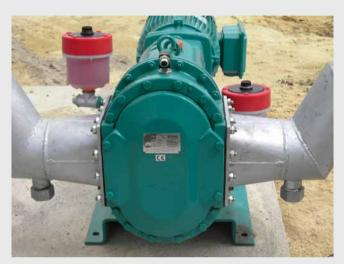
Feed pump for substrate in a biogas plant. Flowrate up to 40 m<sup>3</sup>/h at pressures up to 2 bar.
