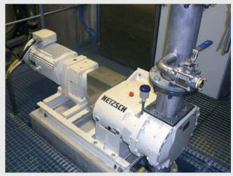
The TORNADO $^{\circ}$  T1 in use in a paper mill. Kaolin tankers are unloaded at 75 m $^{3}$ /h against a pressure of up to 4 bar.
