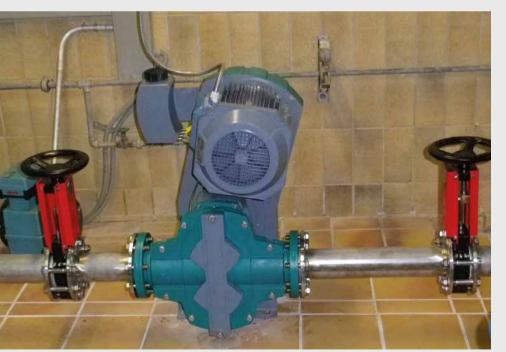
Used in a wastewater treatment plant, the TORNADO $^{\circ}$  T2 pumps sludge with 2% solid content at a capacity up to 18 m³/h against a pressure up to 2 bar.
